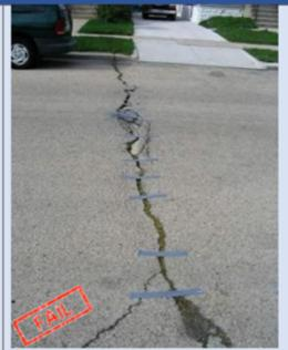
This pavement has a wide crack which is improperly patched.
