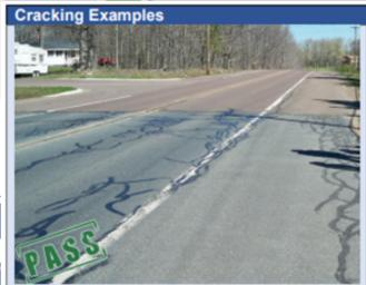
This pavement has significant cracking, but has been patched and should meet the performance measure.
